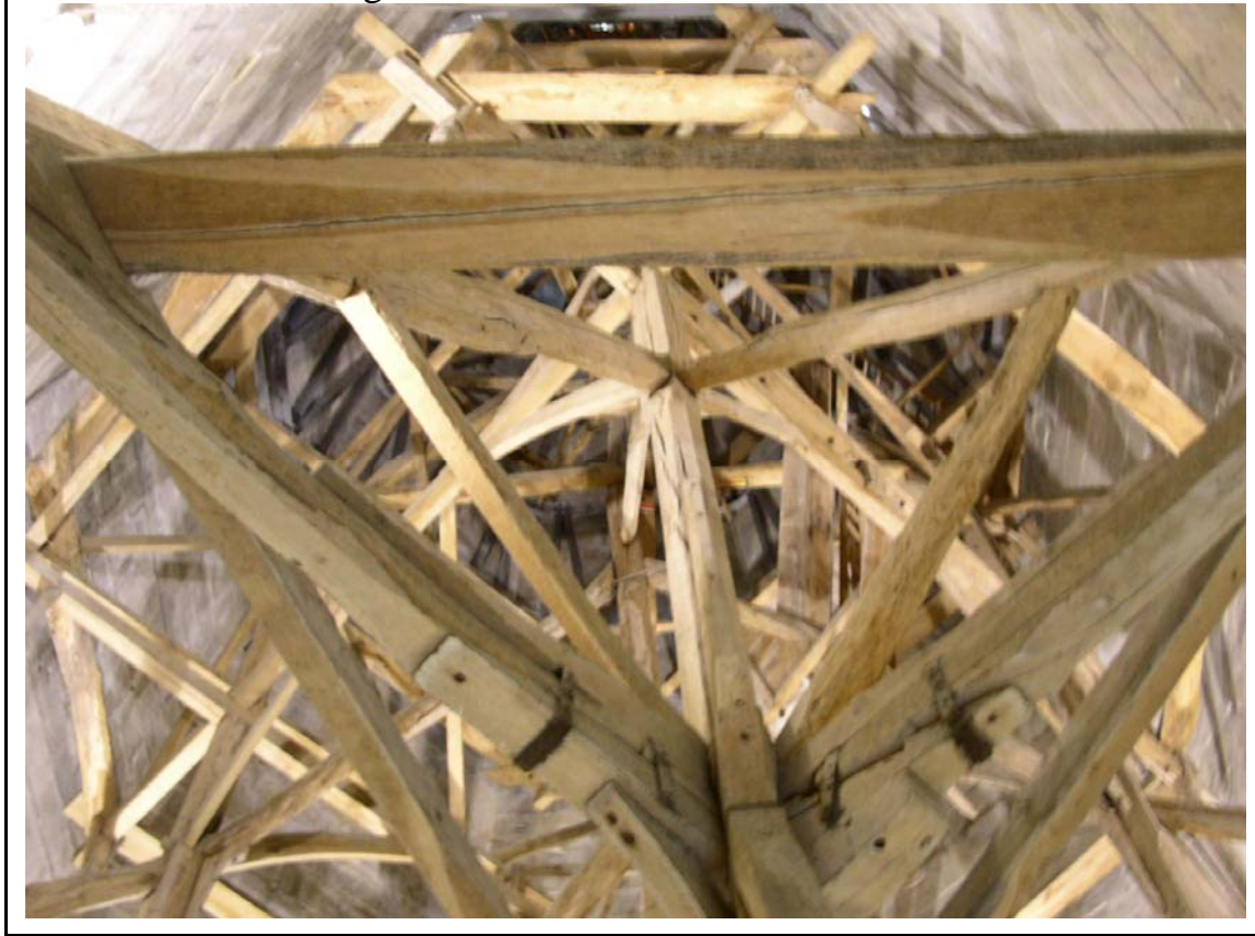
Figure 1. The Scaffold From Below
